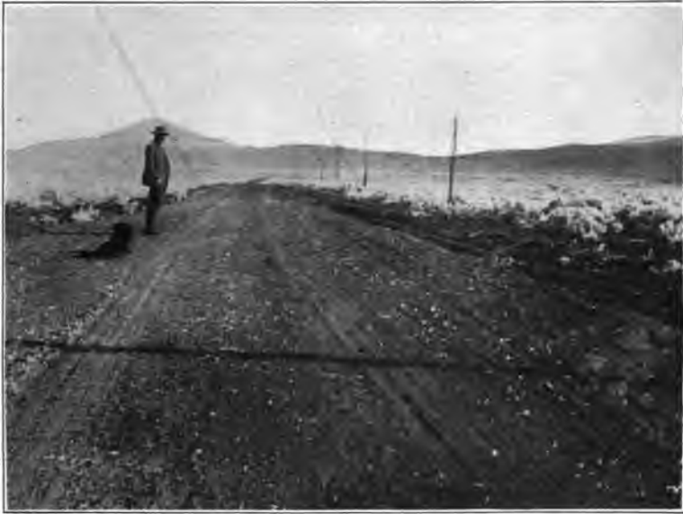
COUNTY ROAD BETWEEN SUMMIT AND PAROWAN, IRON COUNTY.
